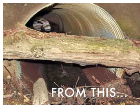
Old Nelson Gulch culvert: 3' wide
