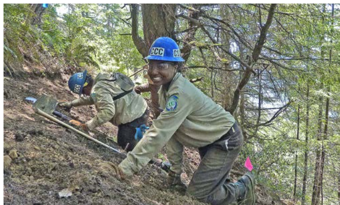
The CCC crew digging into a steep hillside for the trail
