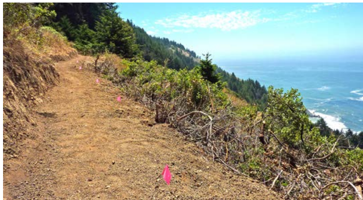
Under construction: a rough cut of the new trail
