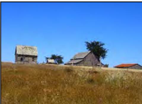
Historic Spring Ranch buildings
