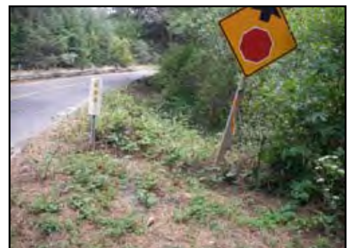
Section of Caspar Beach Trail within the County right-of-way to be improved with Prop 40 funding
