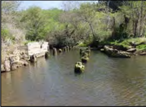
Former Caspar Lumber Mill foundations in Caspar Creek
