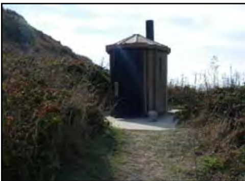
Restroom at Moat Creek
