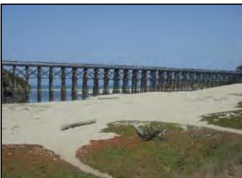
Pudding Creek Trestle, Pudding Creek Beach
